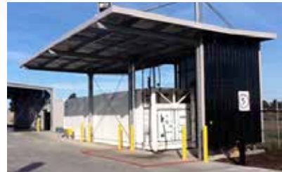
Fleet Refuelling with Canopy Australia
