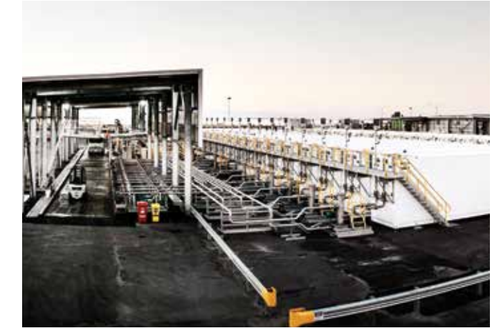
CASTROL BP - 43 x Logitank LSB110 self-bunded tanks, totalling 1.24 million USG of storage for 16 lubricant product
