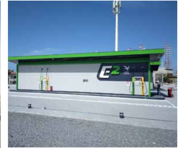
MODULAR FUEL STATION, UAE
